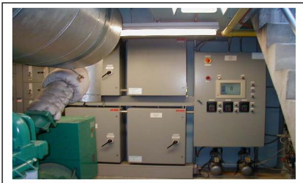
Wastewater Pump Station No. 2 VFD and PLC control panels. Ketchikan, Alaska.
