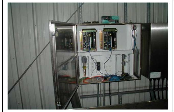
Hot Back-up Allen-Bradley PLC 5 control panel.
