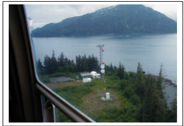
Potato Point Radar Station and Microwave Repeater. Valdez Narrows, Alaska.
